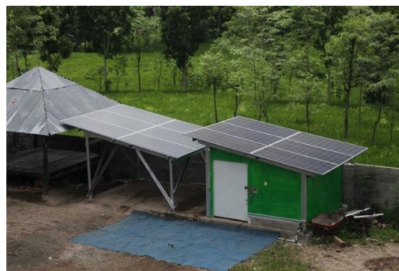
Gambar 3 Instalasi Panel Surya
